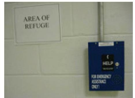
**Figure 6:** Push-to-talk two-way communication box with temporary “Area of Refuge” sign
