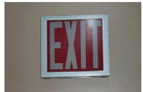
Figure 2: An externally illuminated Exit sign
