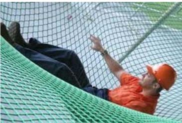
Fig. 6: Netting doesn't help prevent the fall but keeps the fall from causing serious injury.
