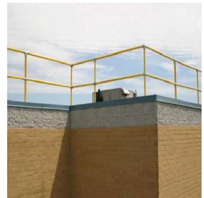
Fig. 1: Guardrails along roof edge
