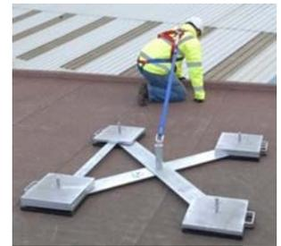
Fig. 5: Fall Restraint System
