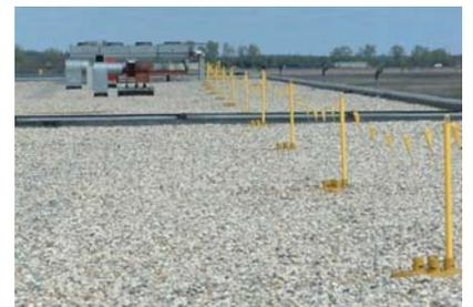
Fig. 7: Warning lines keep workers aware of and away from roof edges.
