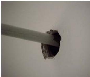
Figure 1: Pipe Poking Through a Fire Wall
