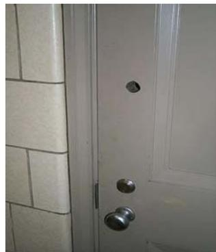
Figure 3: Hole Through Fire Door
