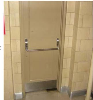
Figure 6: Exit Stairway Door with Panic Bar Hardware
