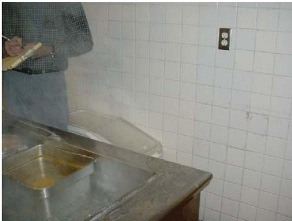
Figure 2 Kitchen outlet not meeting NEC GFCI protective requirements
