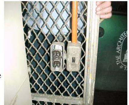
Figure 4: Potentially hazardous outlet with no cover next to switch
