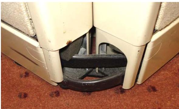
Figure 7: Exposed power wiring at corner unprotected from impact and damage
