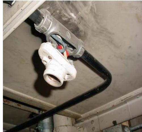
Figure 6: Light fixture not properly secured to mounting with open socket and exposed wiring
