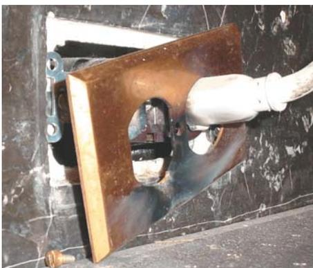
Figure 3: Potentially hazardous burnt outlet with displaced cover
