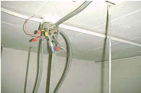
Figure 1: Potentially hazardous electrical junction box without cover
