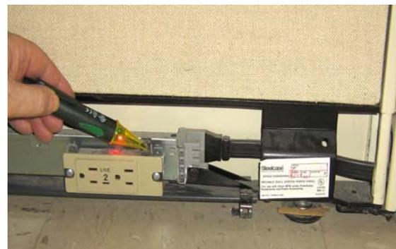
Figure 8: Exposed baseboard electrical supply outlet and service without its cover
