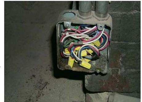
Figure 2: Potentially hazardous wall switch or outlet box without cover
