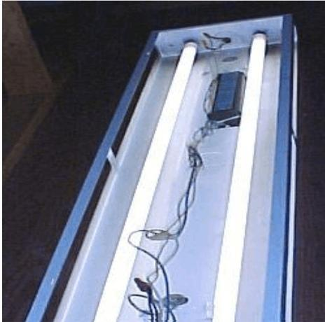
Figure 5: Missing cover on fluorescent light fixture exposes wiring
