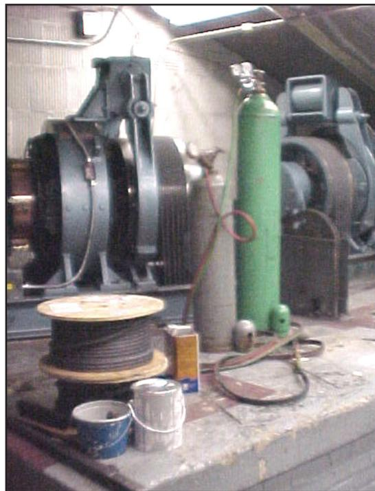
Figure 1: Improperly stored cylinders
