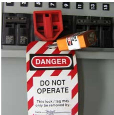
Figure 1: A Proper Circuit Breaker Lock and Tag
