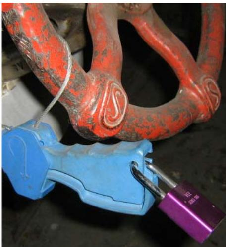
Figure 3: An Untagged LO Device on a Pipe Valve Handle
