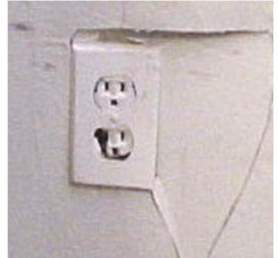
Figure 2: Broken Outlet
