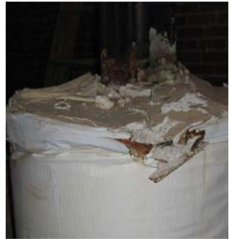
Figure 2: A damaged pipe insulation jacket exposes friable asbestos.
